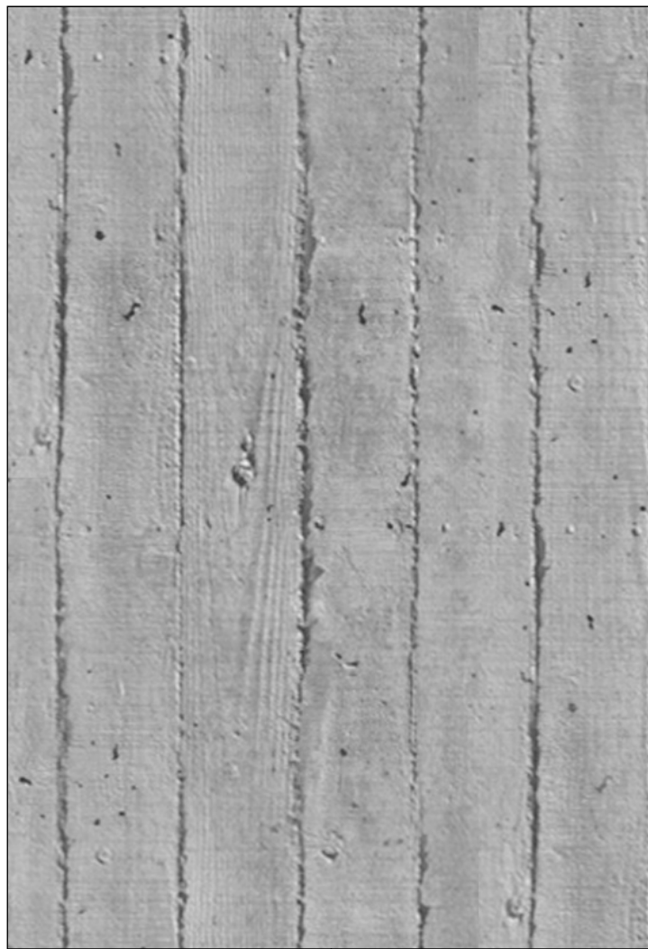
IN-SITU CONCRETE BOARD-MARKED VERTICAL 100MM
